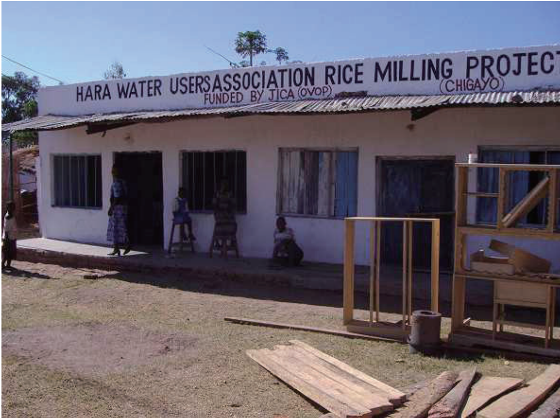
Photo1 Rice mill in Chilumba established by one-village one-product (OVOP) project under JICA
